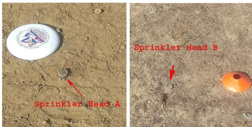
Figure 26. Sprinkler head tripping hazards, November 16, 2021.
