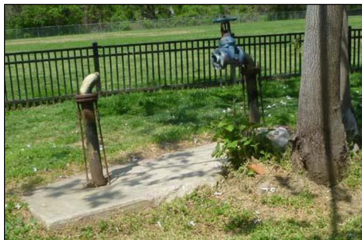
Figure 04. Obsolete 1991 Irrigation Valve.
